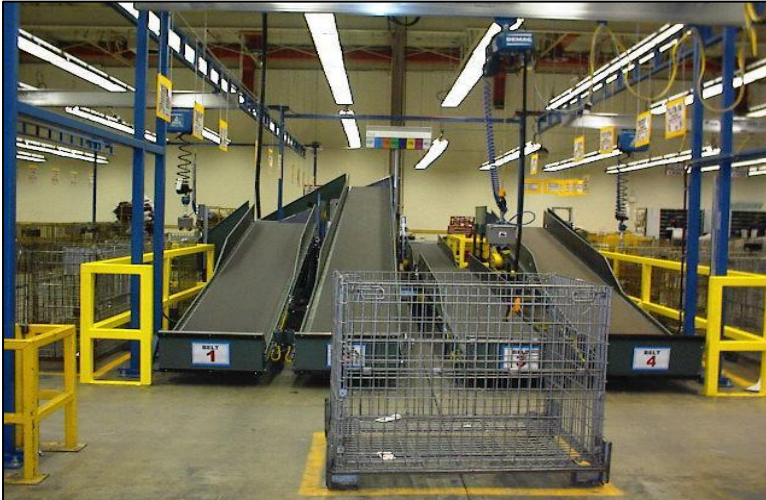
An empty mail container is ready to be taken away from the induction station adjacent to the cell’s four conveyors.
